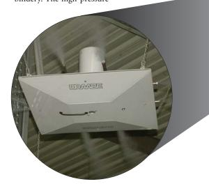
air humidification system uses a pulsating hydraulic flow and titanium nozzles that atomize the water to a micro-fine aerosol. The process is energy efficient and quiet.
