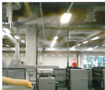
High-pressure atomisers in the print room ensure optimum production conditions
