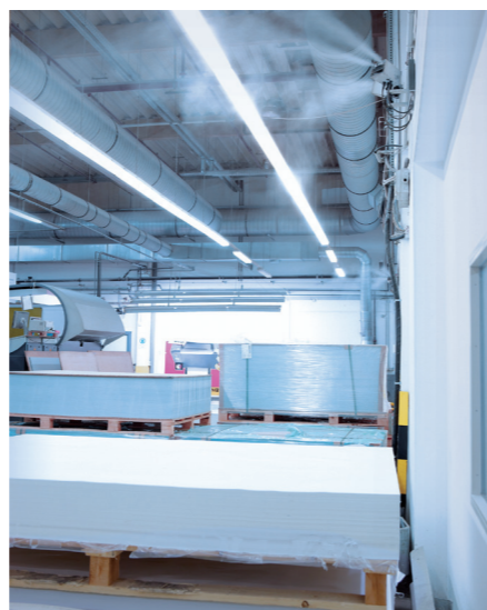
Humidification ensures trouble-free processing of the paper
